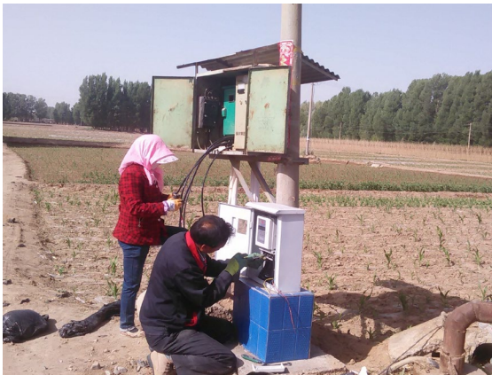
Smart meter installation on irrigation wells
