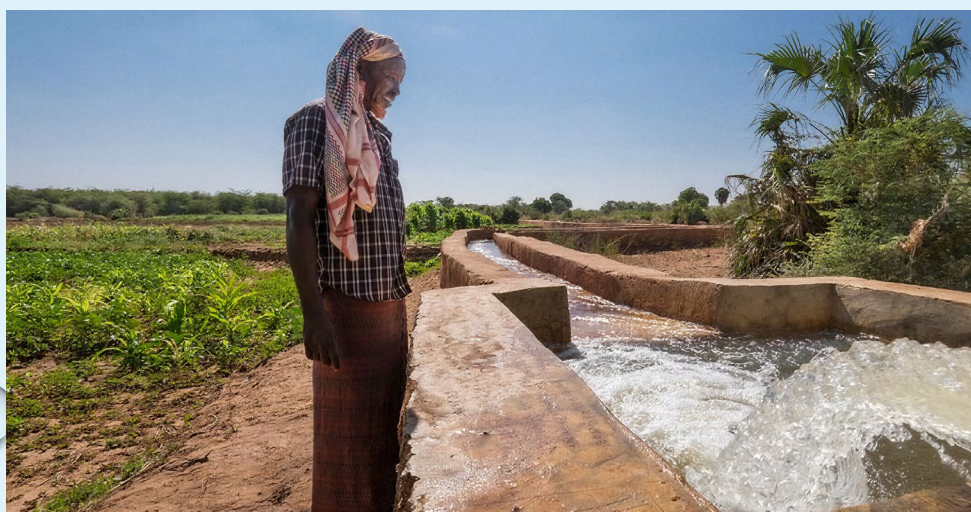
► Figure 6. Irrigation water canal in Unaa Village, Dollow, Somalia © DRC ( SDC , 2021)
