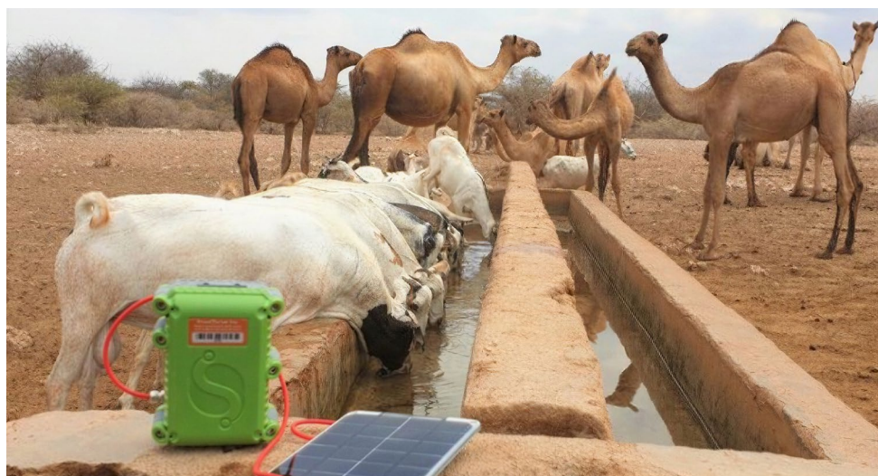
► Figure 4. Livestock watering at Boji Borehole, Isiolo, Kenya (SDC, 2021) © MWA
