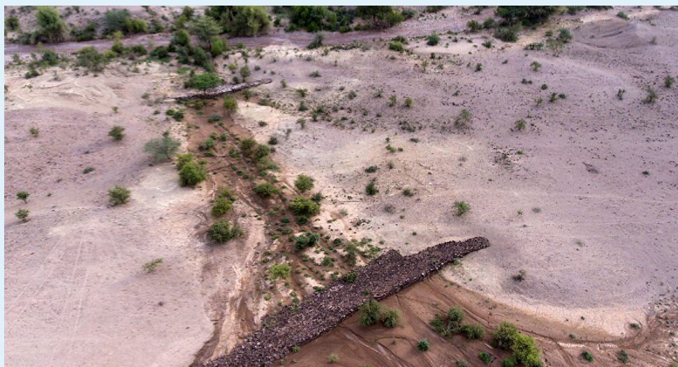
► Figure 3. Dry stone measure from above (GIZ, 2021)
