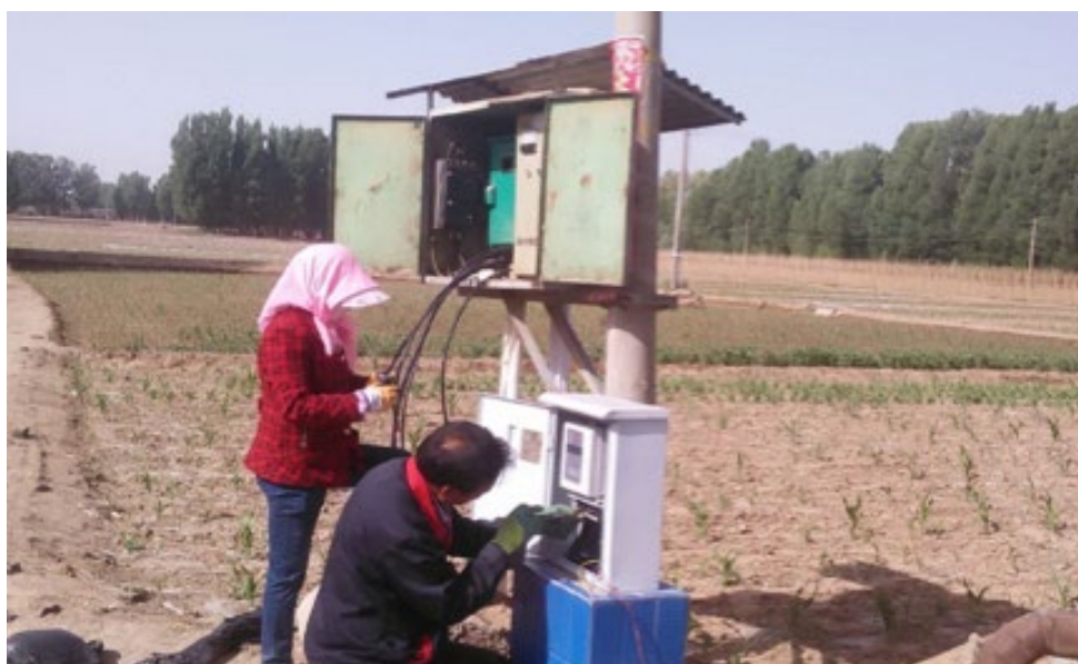
► Figure 5: Installing smart meters on an irrigation well in China ( Wang, 2025 ).
